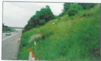
Figure 2. Cutting on the M69 where vegetation may have stabilised sections next to the failure.
