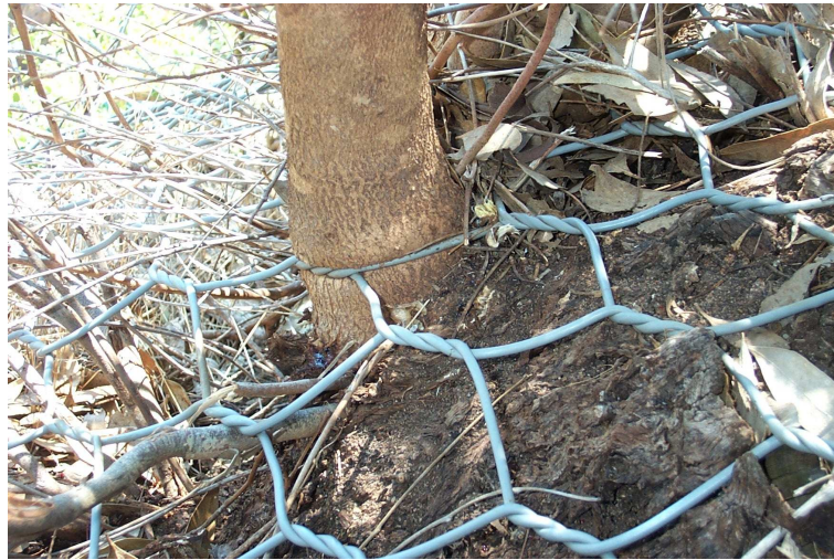
Figure 9: Young eucalypt growing on a rockface through the aperture in draped mesh.
