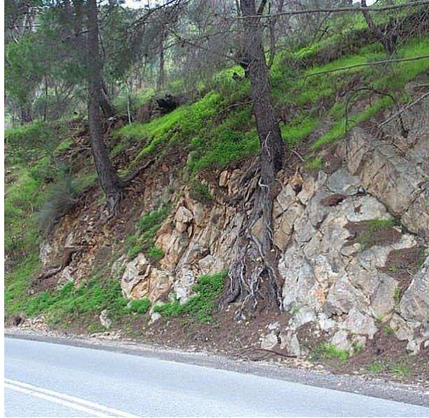
Figure 2: Mature pine trees growing on a 7 m high rock slope, 10 m from the site of a 5 m 3 toppling incident.
